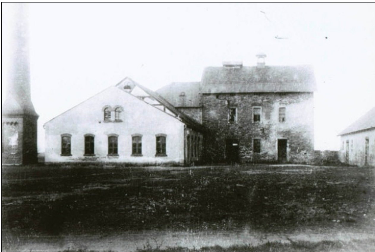
Fig. 9: The building to the right, which did not survive, contained the water powered whim (Reymann, ca. 1900).
